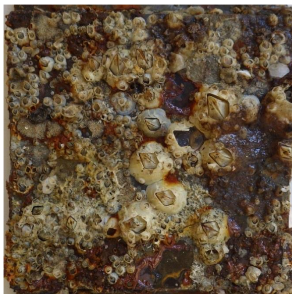
Figure 10: Corrosion and biofouling on a mild steel panel protected with a “user applied” anticorrosive coating.
