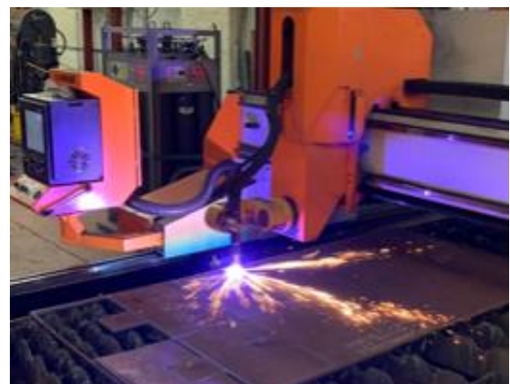
Frame sections being fabricated: end flange plates being cut-out of sheet steel.
