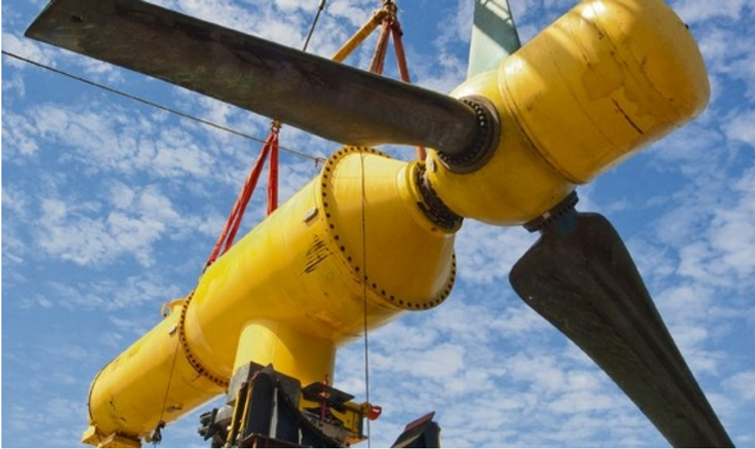
(a) The 500KW DEEPGEN III being lifted by crane barge (not in scene).
