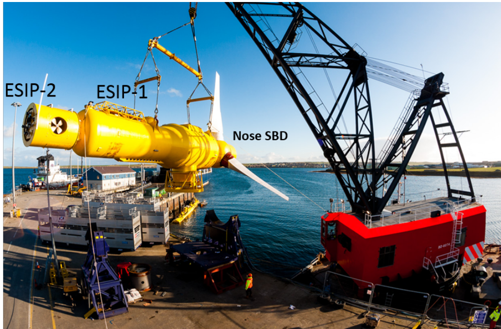
Figure 3.6: Photograph of DEEPGEN IV being lifted by crane barge prior to deployment. Locations of the UoE instrument platforms, ESIP-1, ESIP-2 and the nose SBD identified.
